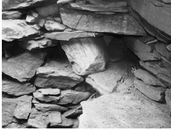
Fig. 5a. Cavities in the west wall and used as niches
