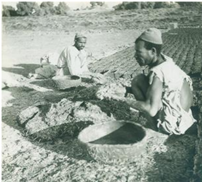
Figure 39 New Gourna, brick making, from the archive of Hassan Fathy AUC 99
