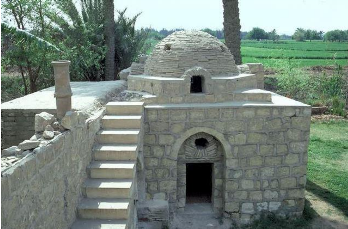
Figure 18 Fouad Riad House Giza, Egypt
