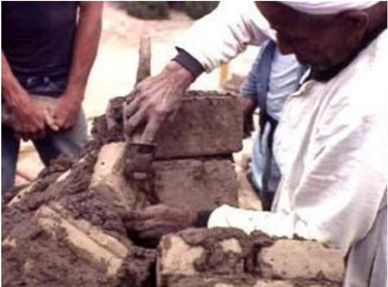
Figure 41 a construction of a mud brick dome 103
