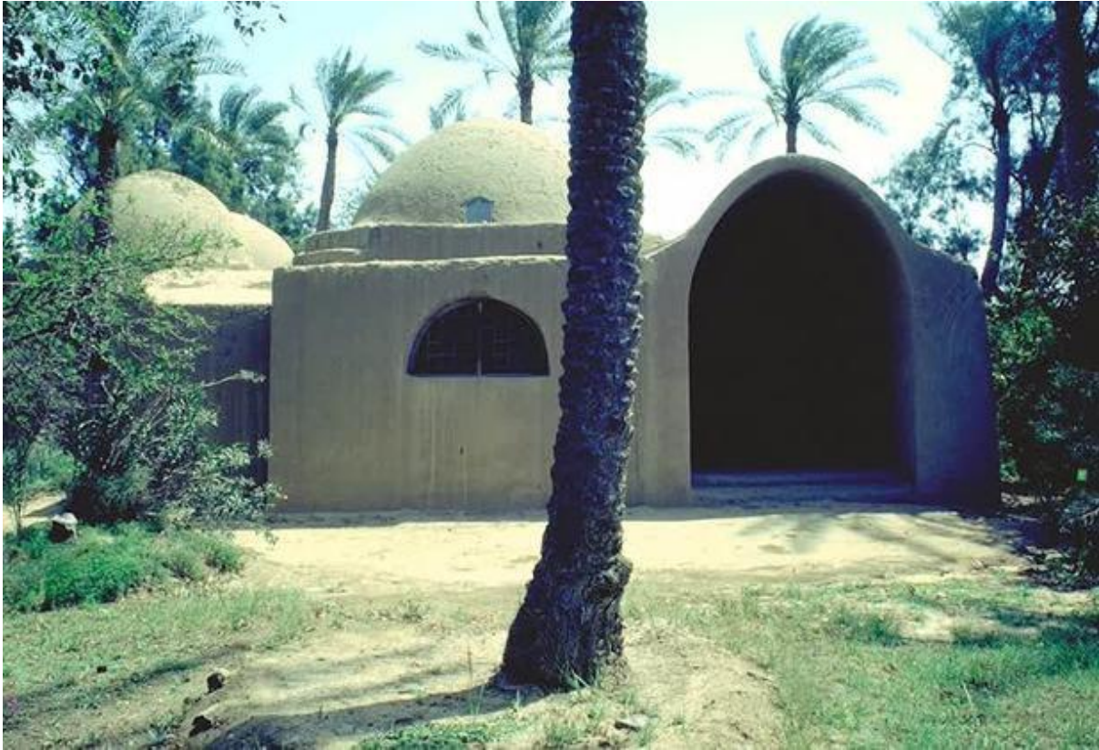
Figure 9 Hamed Said House Cairo, Egypt
