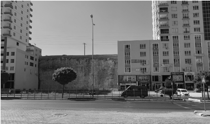
18 19 20 Figure 5.3: New Settlement, built without regard for the local topography 21 (Source: author's photograph)
